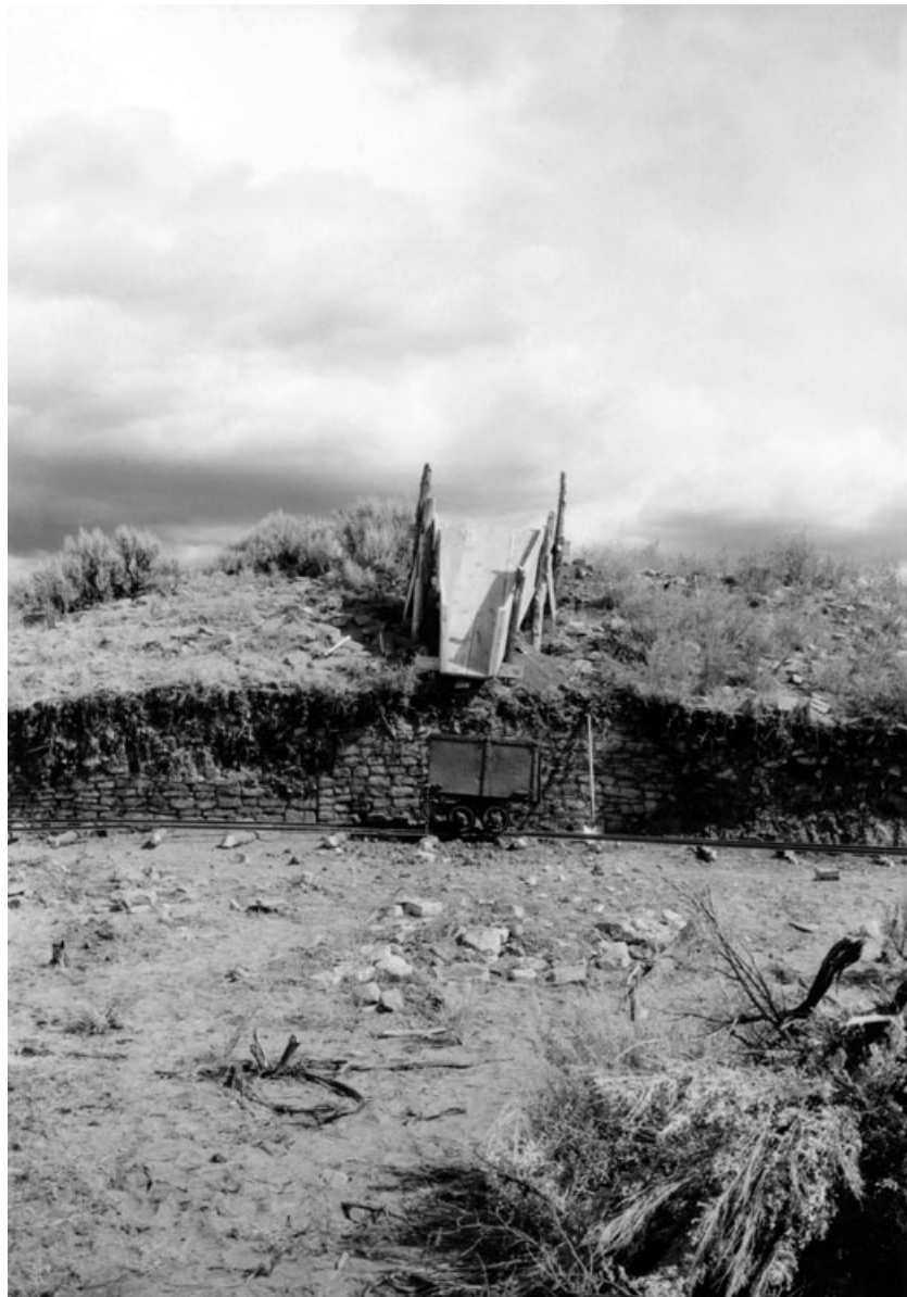
FIGURE 2. Mining chute, car, and track used to quickly remove overburden from south end of Lowry Ruin during the 1930 field season. (Negative No. CSA76312; courtesy of the Field Museum)
